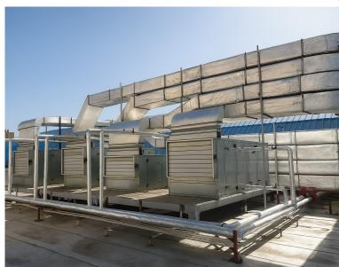
Depending on the needs of the consumer, the device has a cooling, pre-heating and post-heating converter.
